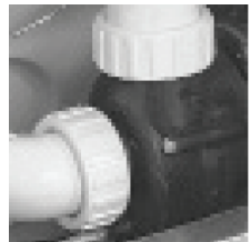
Vent air by slightly opening pump unions.
